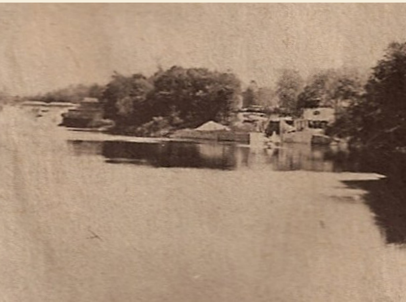
The terminus of the Black River Canal into the navigational portion of the canal below Lyons Falls (High Falls). Credit: Lyons Falls History Association's photo library.
