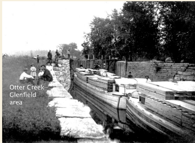
The Otter Creek lock on the navigational portion of the Black River Canal. Credit: Lyons Falls History Association's photo library.
