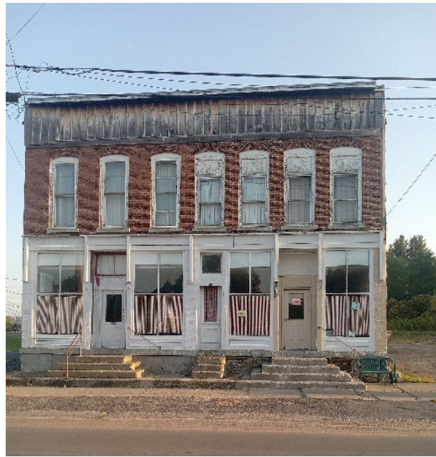
7090 W. Main Current Condition
