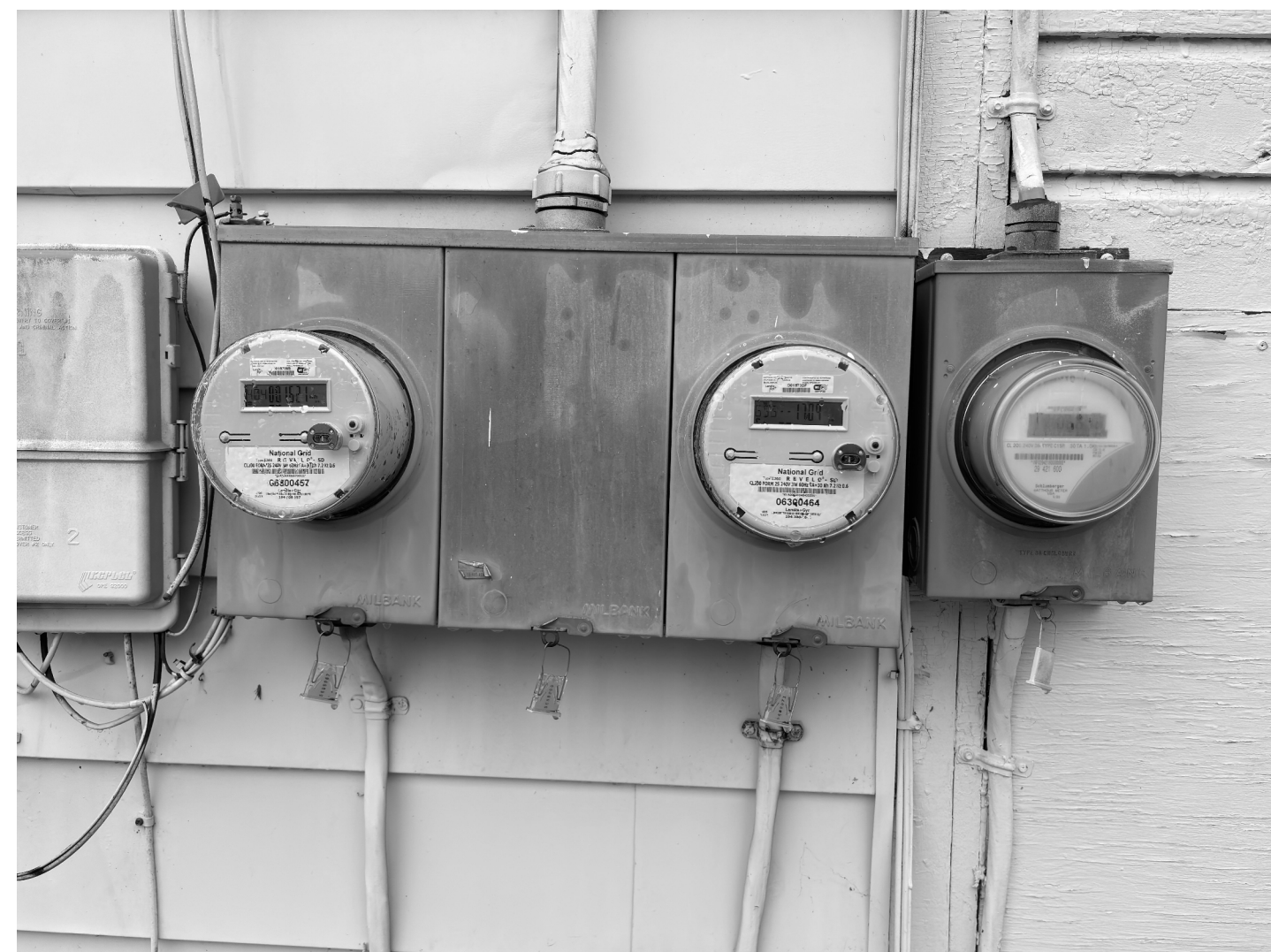
PHOTO #4 - EXISTING UTILITIES
