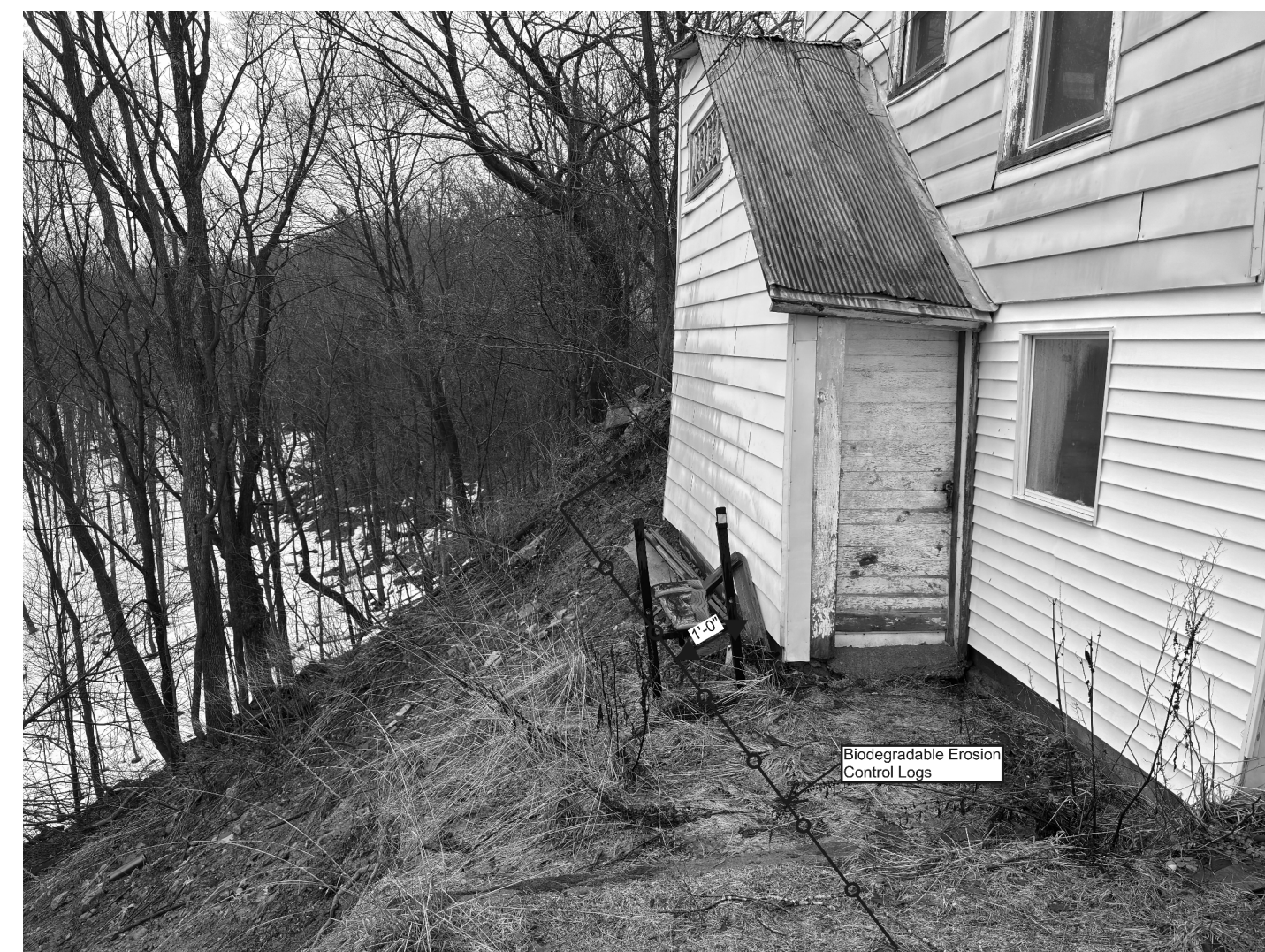
PHOTO #5 - EXISTING SITE - BACKSIDE OF PROPERTY
