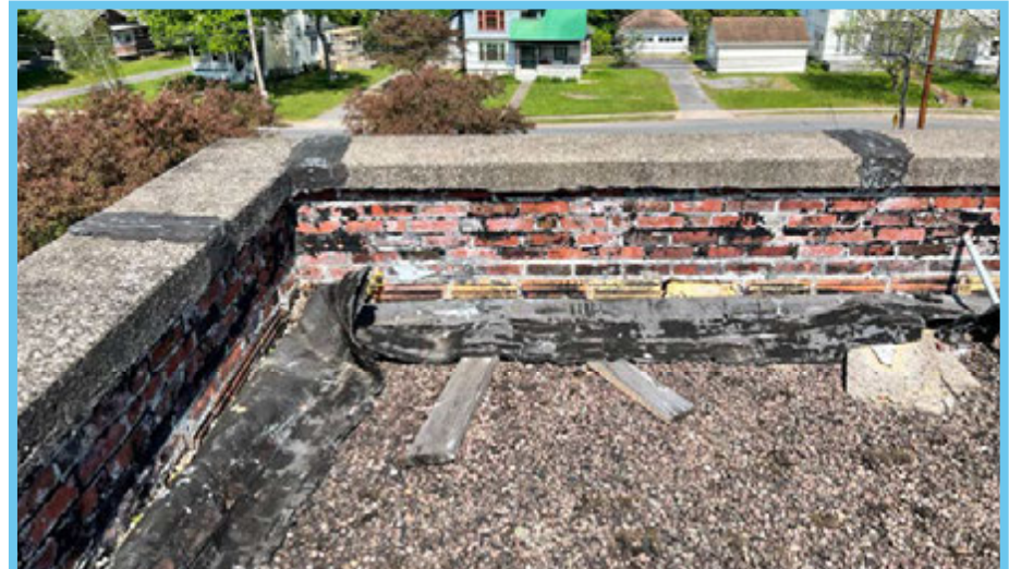
LYONS FALLS ELEMENTARY SCHOOL - DEBONDED ROOF FLASHING AT MASONRY PARAPET / PHOTO SOURCE: DANC
