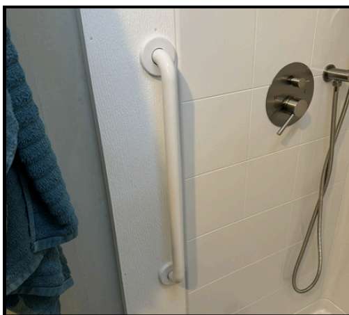
Grab bar installed into a shower unit
