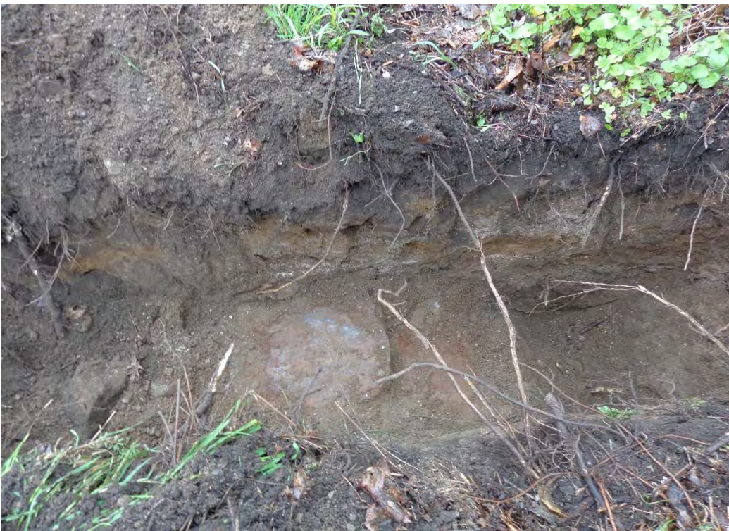
Test Pit TP-2 view of manway for underground heating oil tank
