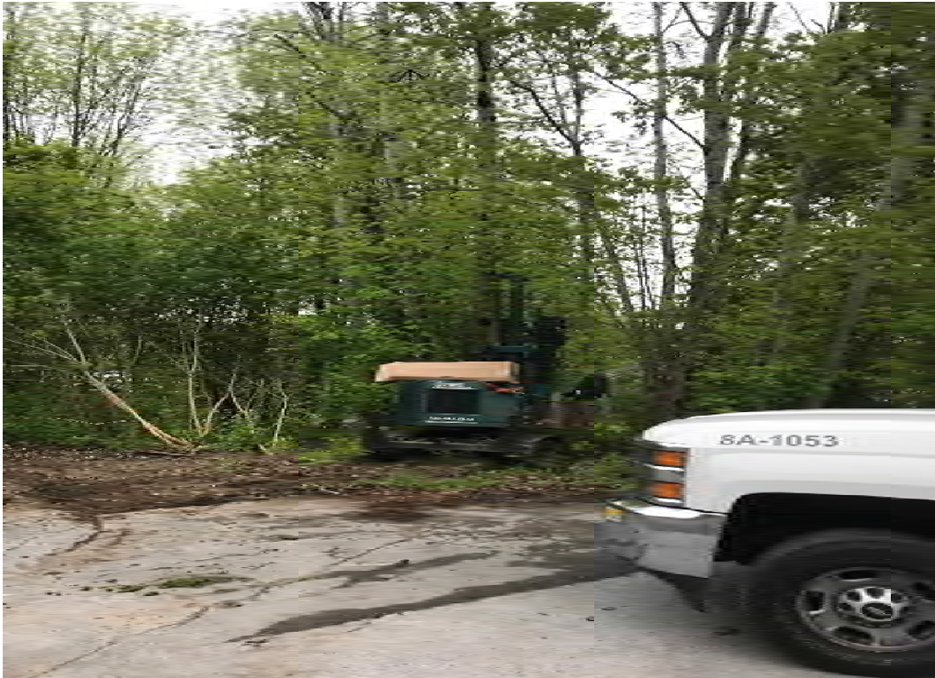
Installation of soil boring SB-5 / monitoring well MW-1 (view looking north)
