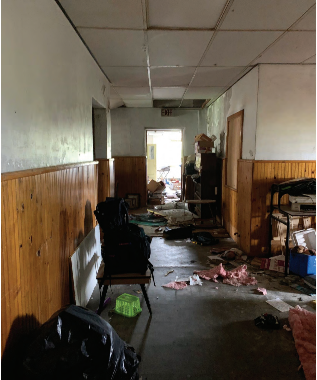
Second floor hallway.
