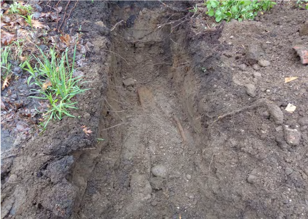
Test pit TP-1 view of top of underground heating oil tank
