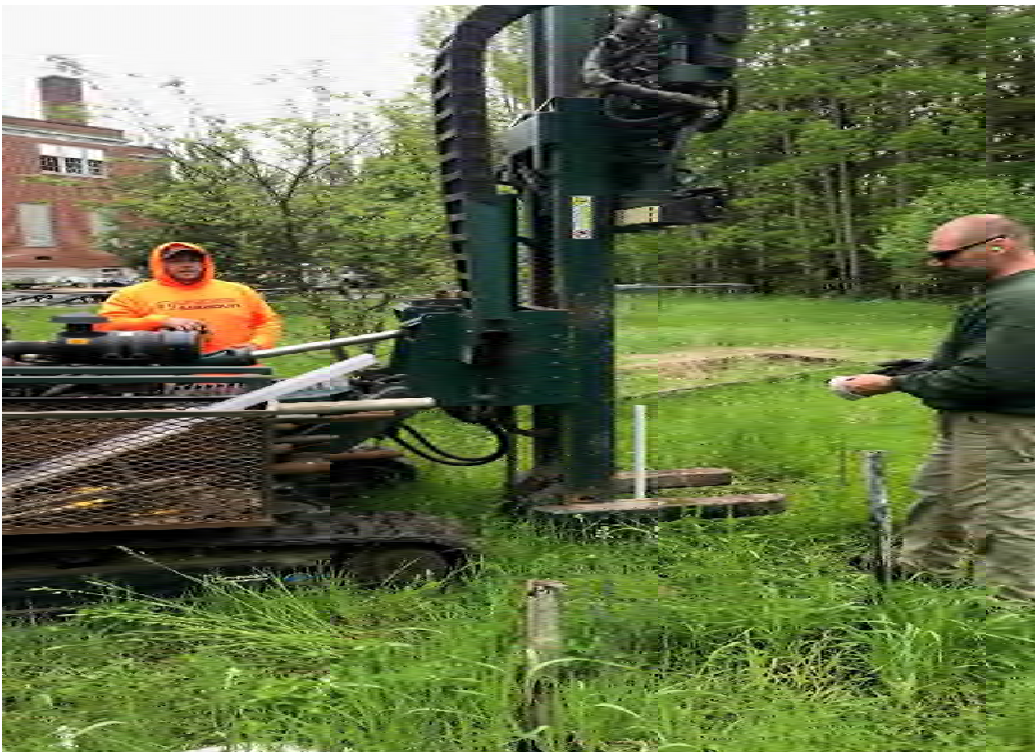
Installation of SB-8 /MW-2 in rear yard area view looking north)
