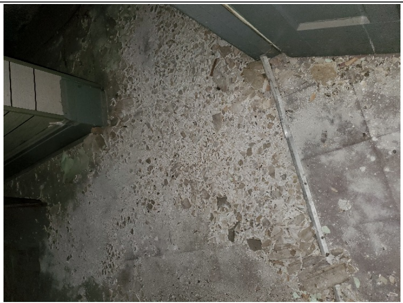
Material 23020-001 9" x 9" Floor Tile This material is present beneath non-ACM plaster debris and guano.
