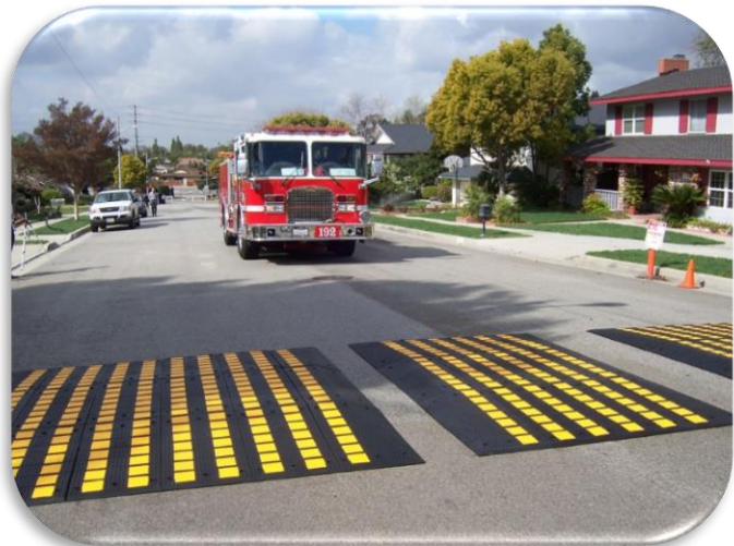
Speed Cushion in use by Firetruck; Image Source: https://nacto.org/publication/urban-street-design-guide/street-design-elements/vertical-speed-control-elements/speed-cushion/
