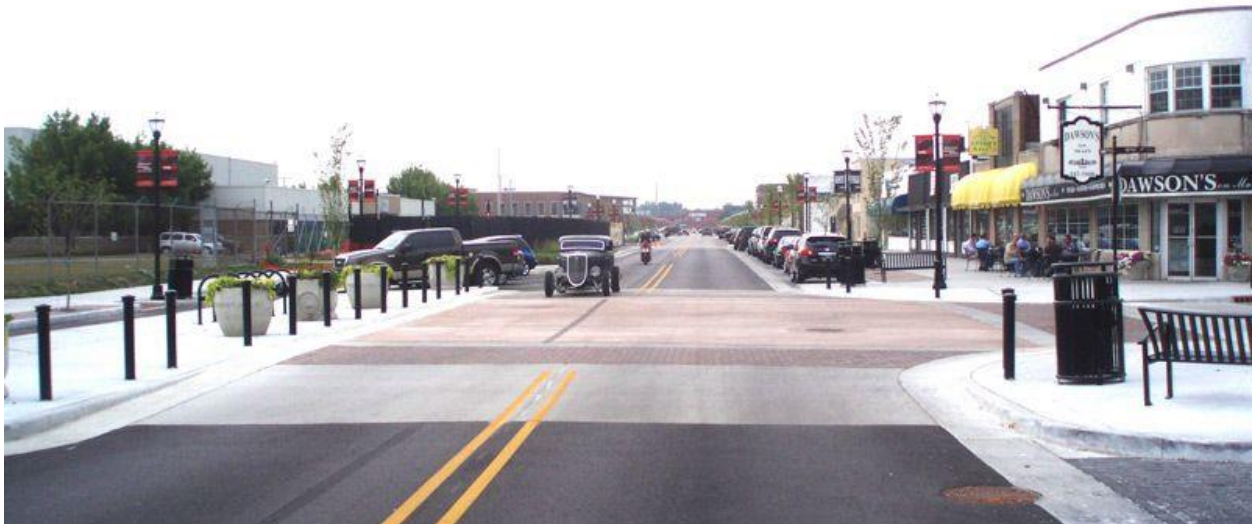
Raised Intersection; Image Source: https://goshenindiana.org/blog/intersection-closure-jackson-and-9th-streets/
