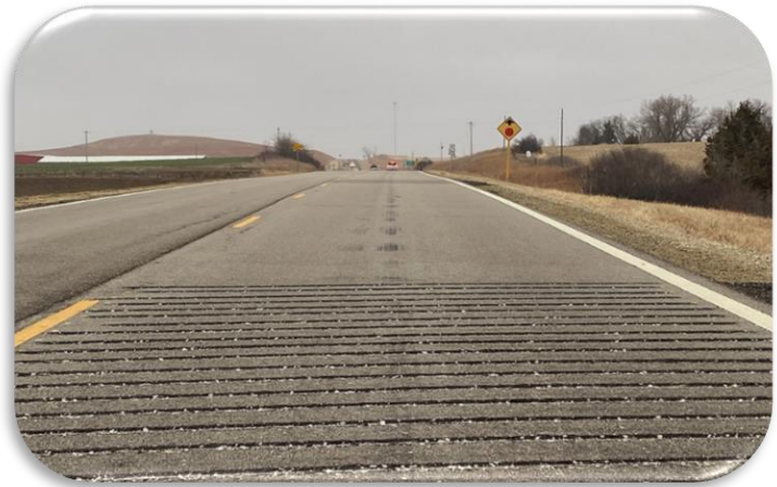
Rumble Strip; Image Source: https://www.backroadsnews.com/news/rumble-strips-installed-intersection-us36
