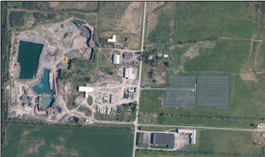
This image depicts the location of a constructed 2.9 MW solar project in the town of Hounsfield 44 . The project was sited in an 'Industrial' zoning district adjacent to a mining operation and a manufacturing operation.
