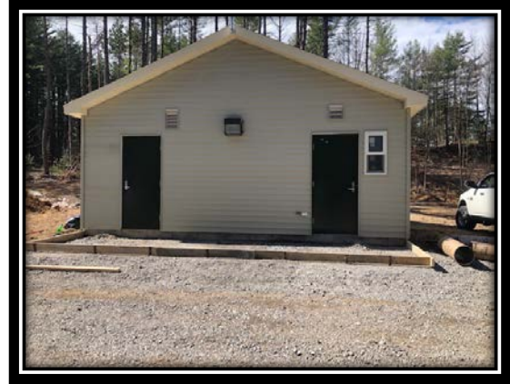
Picture: Town of Watson Treatment Building Water District #4 Ext. #1
