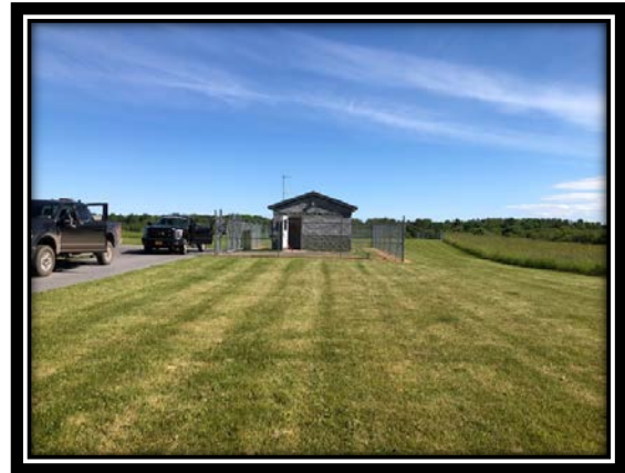
Picture: Town of Martinsburg Treatment Building Water District #1
