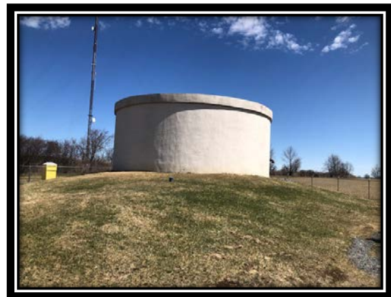
Picture: Town of Lowville Drinking Water Storage Tank Consolidated Water District #1
