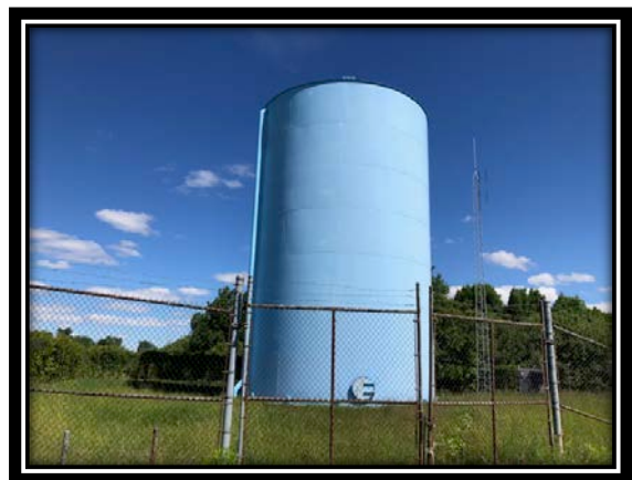
Picture: Town of Denmark Drinking Water Storage Tank
