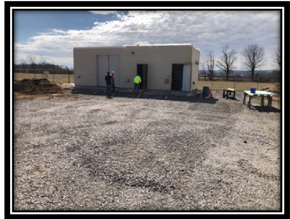
Picture: Town of Lowville Treatment Building Consolidated Water District #1
