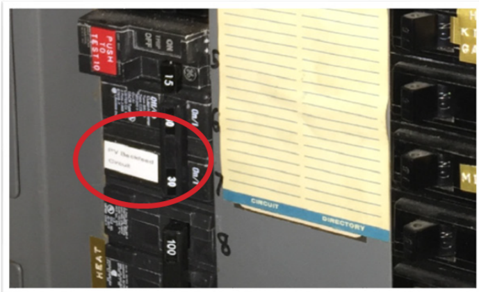
Photo 3: Working clearance not maintained: NEC 110.26
