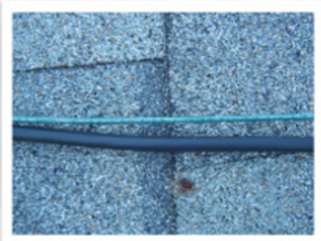
Photo 8: Source circuit conductors in contact with roof: NEC 338.10, 334.30
