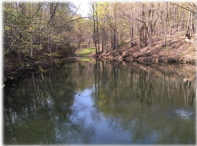
Picture: 1,000,000 gallon reservoir
