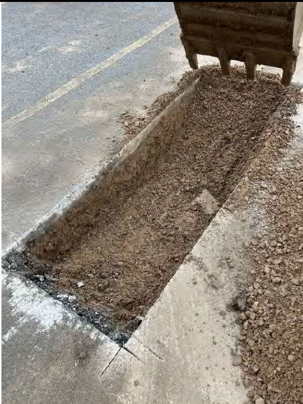
Test Pit #2 Pavement Section and Geotextile Fabric
