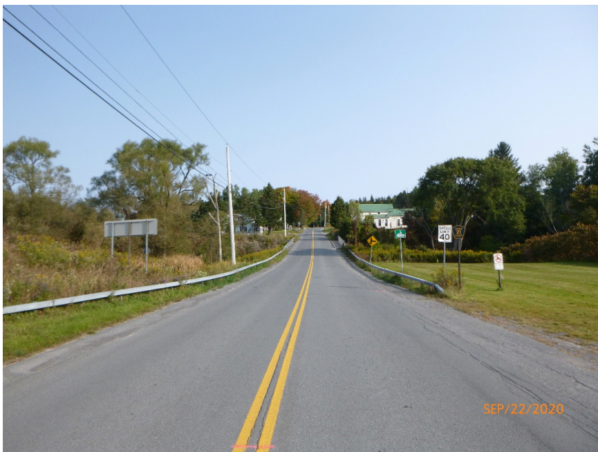
END APPROACH (LOOKING NORTH)
