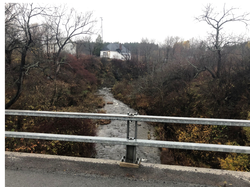
DOWNSTREAM FROM BRIDGE
