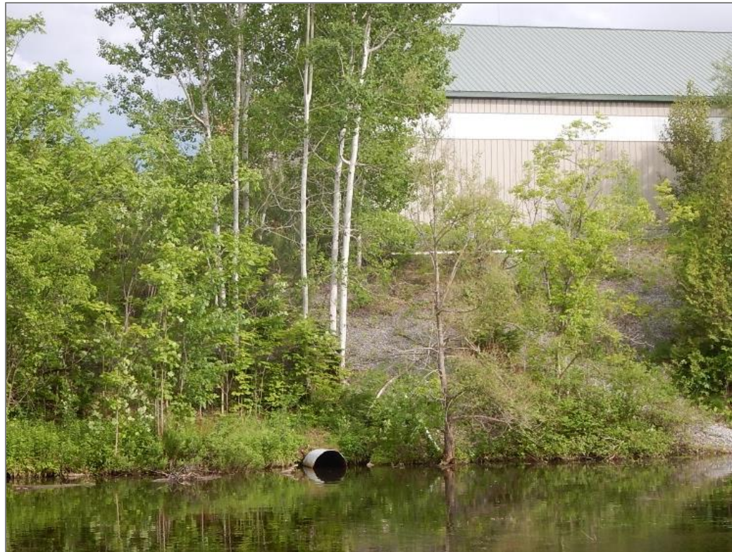
Figure 4 Storm Sewer Outlet into the Turning Basin
