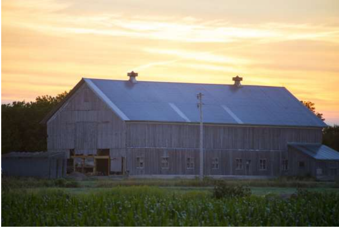
Former Dairy Barn, Lowville, NY. Photo by Eric Adsit
