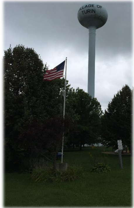
Picture: 200,000 gallon storage tank
