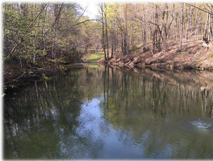
Picture: 1,000,000 gallon reservoir
