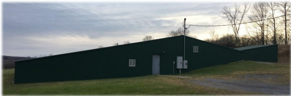
Picture: Water Filtration Plant
