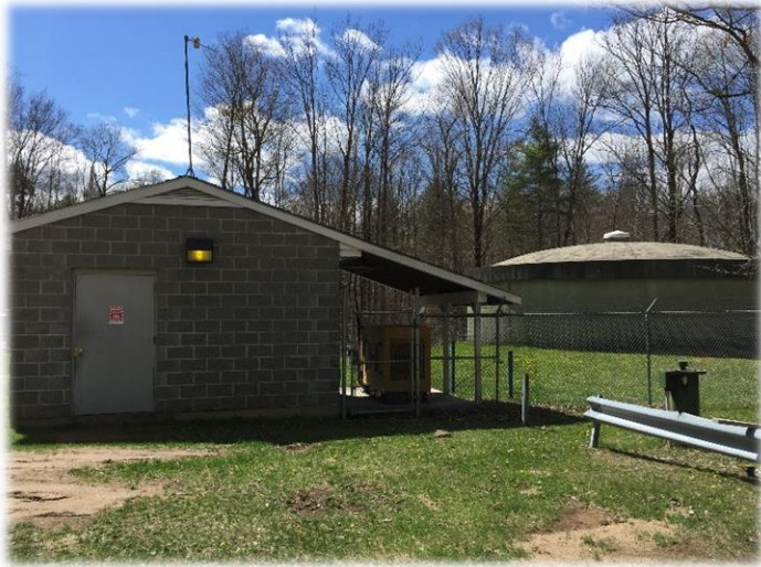
Picture: Burnt Shanty Road well, chlorination, and storage tank site
