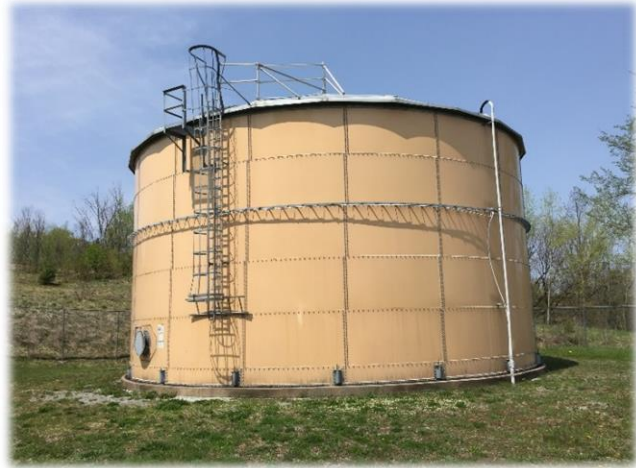
Picture: Rugg Road 325,000 gallon storage tank
